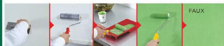
Step 1: Apply the texture paint. Step 2: Before it is dry roll the roller. Step 3: After it is dry, paint the color. Step 4: Painting color.
